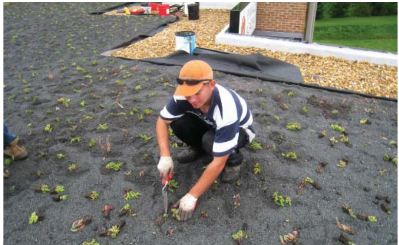
Planting “plugs” on green roof of Mildred Park Center
